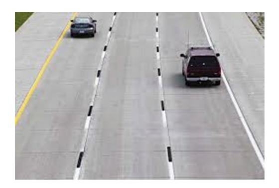
This would include installing black contrast striping over the current roadway markings on eastbound and westbound I-264 to improve visibility in areas where pavement is lightly colored or subject to glare from the sun. High-visibility striping helps drivers navigate the interchange and can reduce unnecessary or last-minute lane changes.
