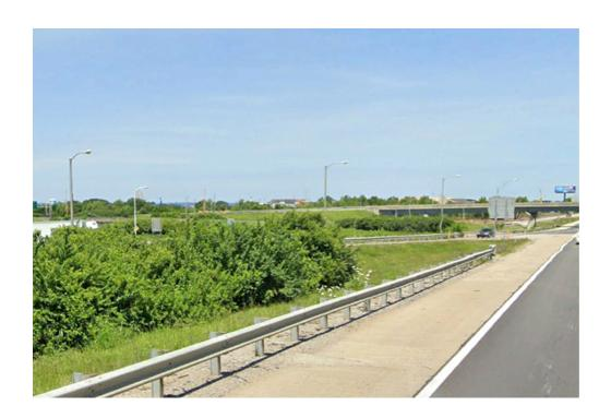
This would include upgrading the existing guardrails within the interchange to defined KYTC standards and the latest research on roadside barriers to reflect the types of vehicles and conditions most likely present on the roadway. This provides improved protection in the event drivers depart the roadway.
