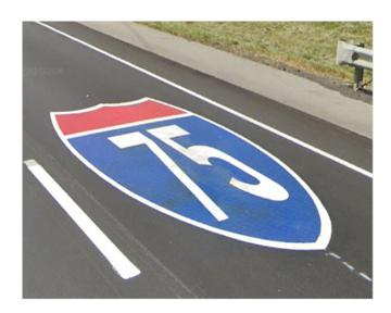
This would include installing markings, also known as route shield pavement markings or 'pavement tattoos,' directly on the roadway to identify which lanes drivers should choose to reach their desired destination. Pavement tattoos help drivers keep their eyes on the road and can reduce unnecessary or last-minute lane changes. The pavement markings would not replace but aid in overhead or side panel signage.
